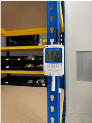
Rack / Warehouse (Cobalt XS / Smart Hygro Temperature and relative humidity Sensor)
